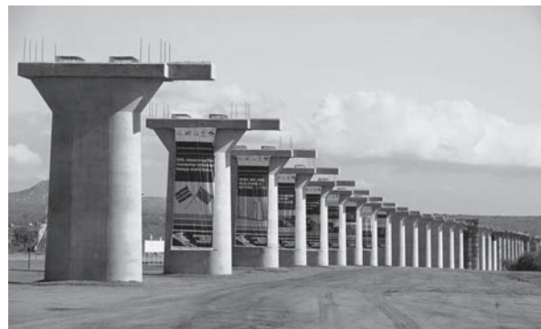
Note : The 1987.7 meters long Tsavo Super Bridge, with the highest point of 35.1 meters being constructed by China Road and Bridge Corporation (CRBC) will run over the Tsavo River and the existing meter gauge railway.
